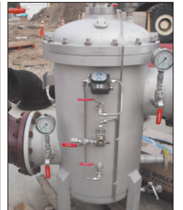
Figure 4, left, shows the cartridge filters upstream of the LPRO membranes. The 5-µm cartridge filters represent the last screening step before water reaches the membranes.
